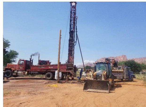
Cluff Drilling setting up on Well 22
