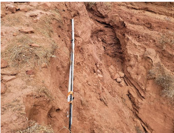
A temporary splint to keep the line from breaking.
