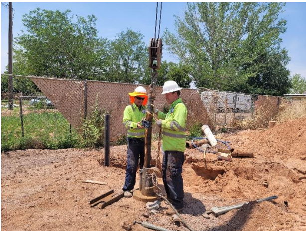
Nathan and Ralph lowering the drop pipe in the new well 4.
