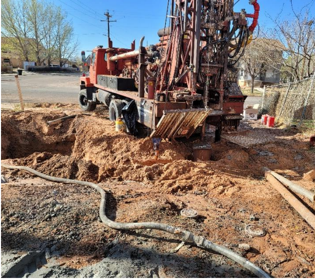
Installing casing for Well 4
