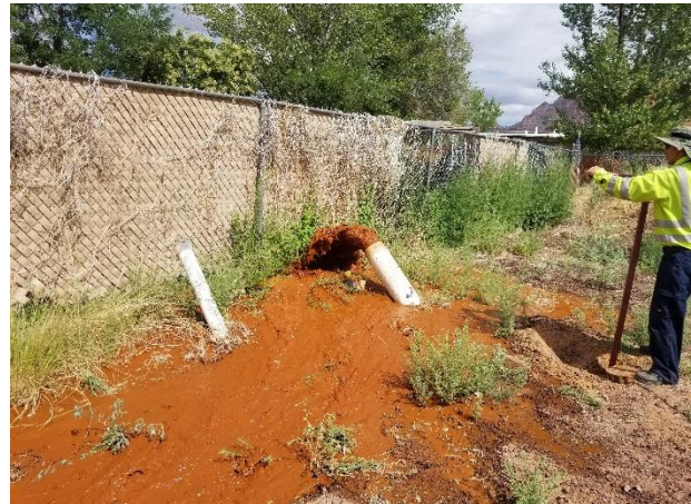
Flushing the collection lines
