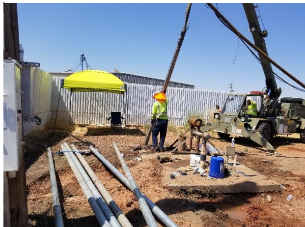
Lifting new pump and motor for Well 17
